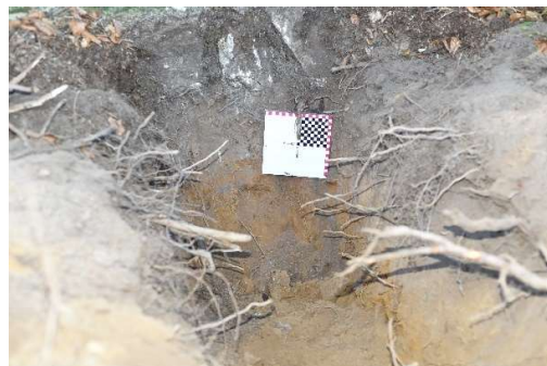
Photo 2 – TP2 Pit at Burial Ground – Scrub roots noted, but no roots under-passing wall
